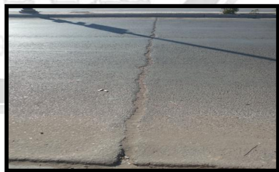
Transverse cracking
