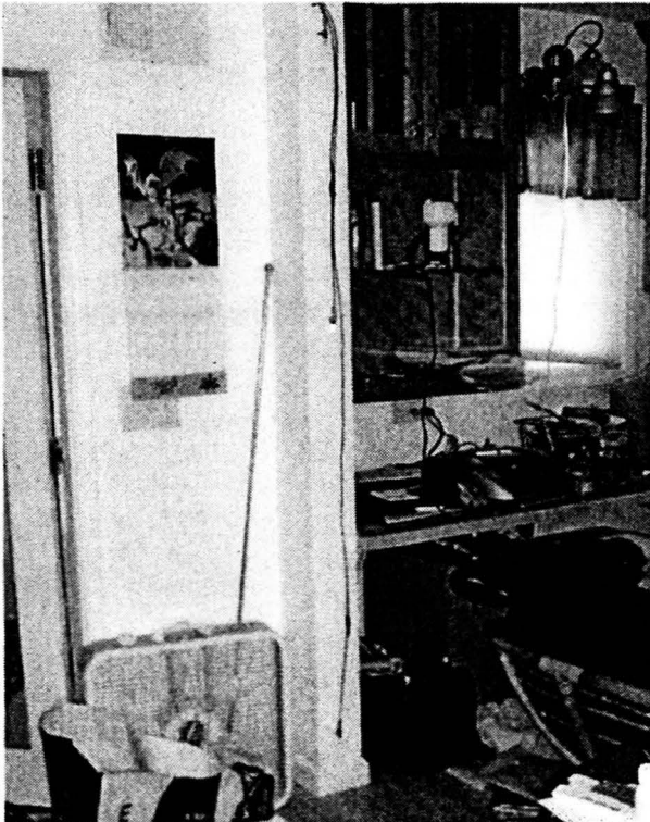
These are the temperature and humidity sensors in the 2002 house.
