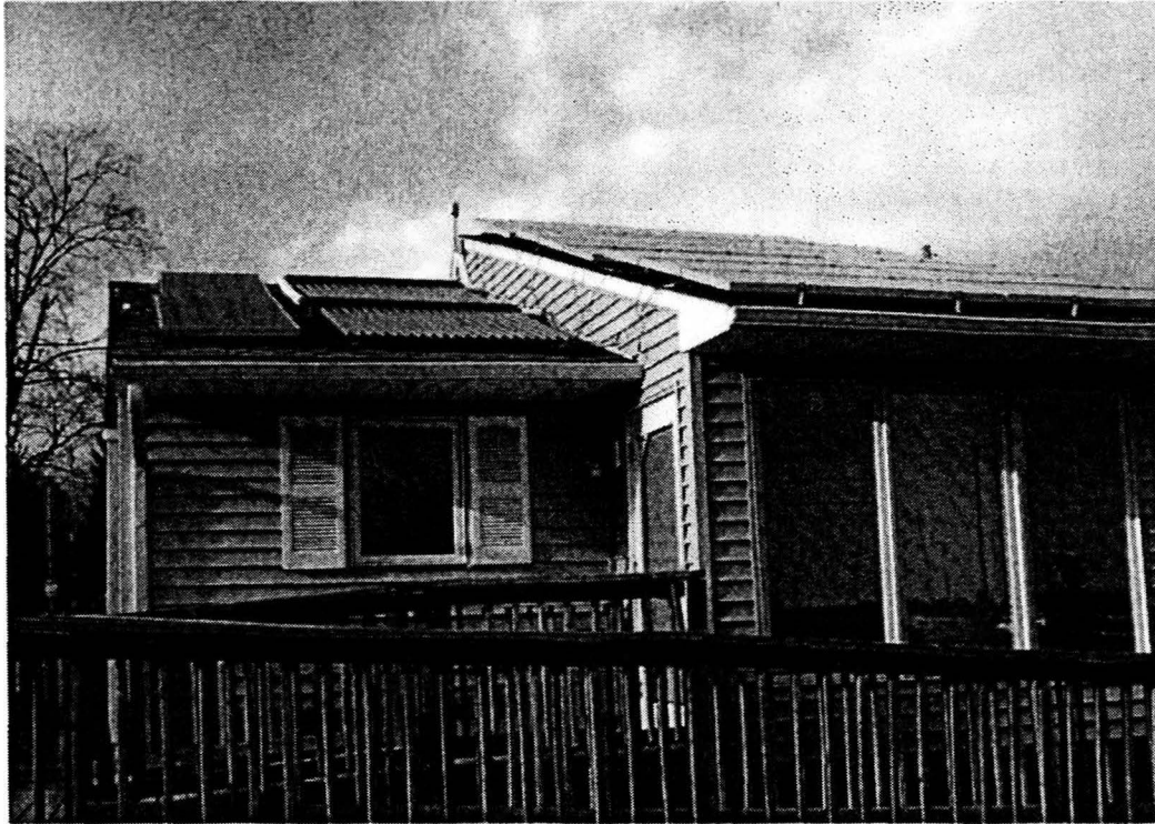
This is a photo of the 2002 UMR/RTI competition solar house. The pyranometer is in the middle of the two modules, sticking up above the rest of the house.
