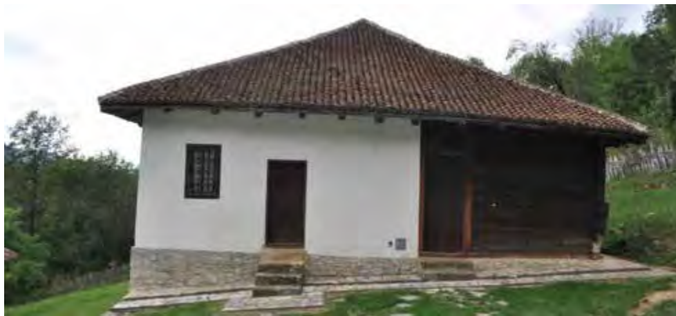
Fig. 1. The house of Živojin Mišić in Struganik, an example of 19 th century vernacular architecture in Serbia (own photo)
