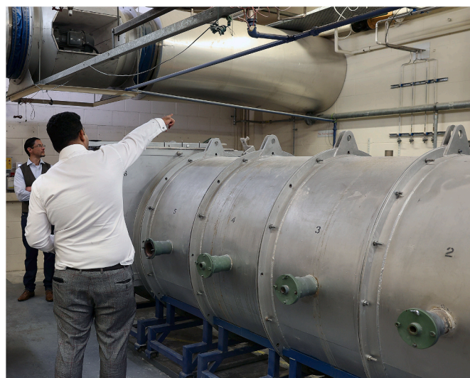
Fig. 5. Commissioning of a 1.5MW unit operating with ammonia blends for steam production. Cardiff University Centre of Excellence on Ammonia Technologies.
