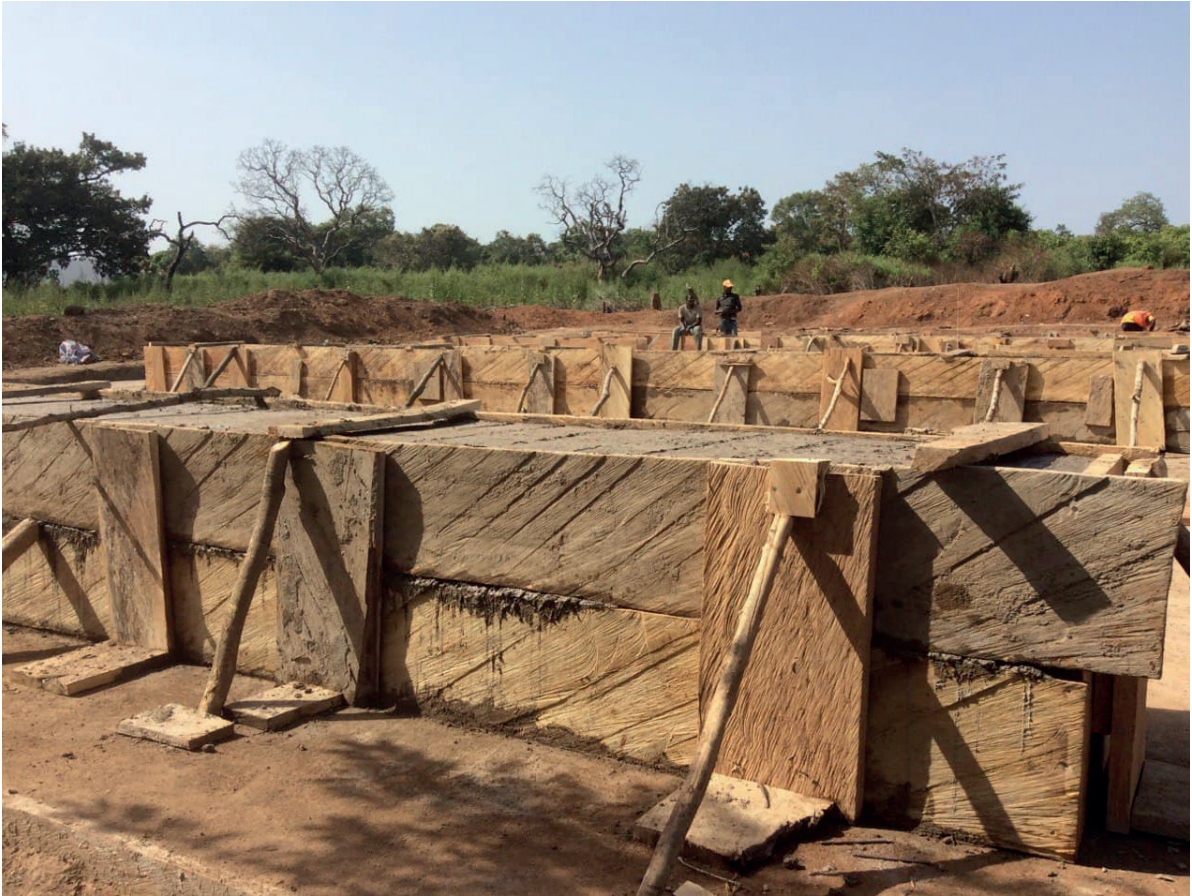
Figure 35 - Image of the construction process. Footings and basement
