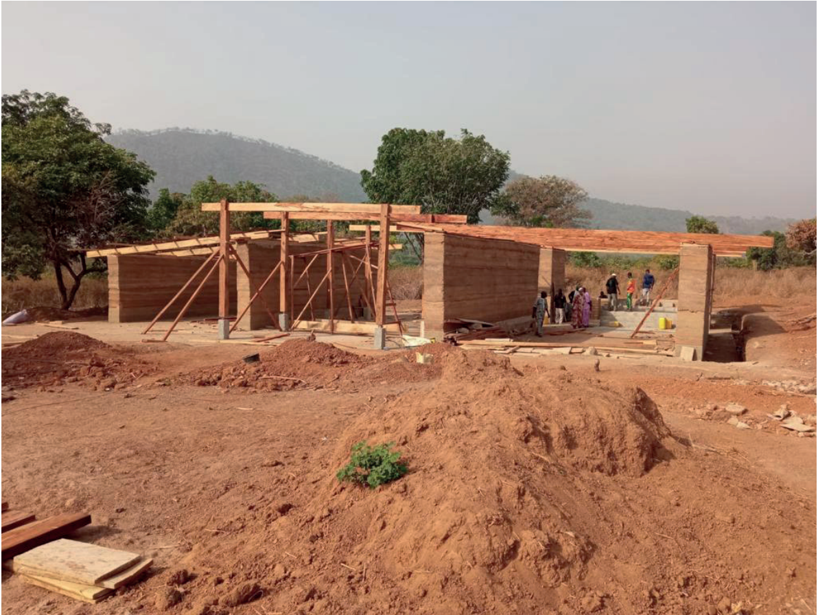
Figure 36 - Image of the construction process. Wood bond beams
