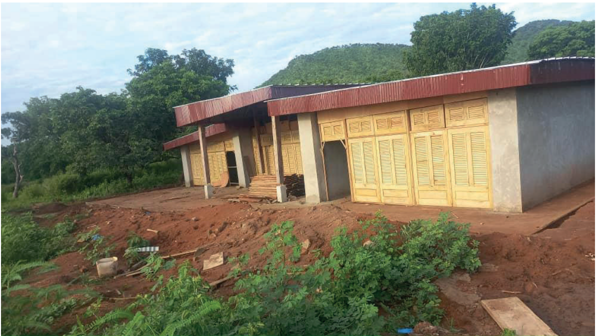
Figure 37 - Image of the construction process. Lasts additions
