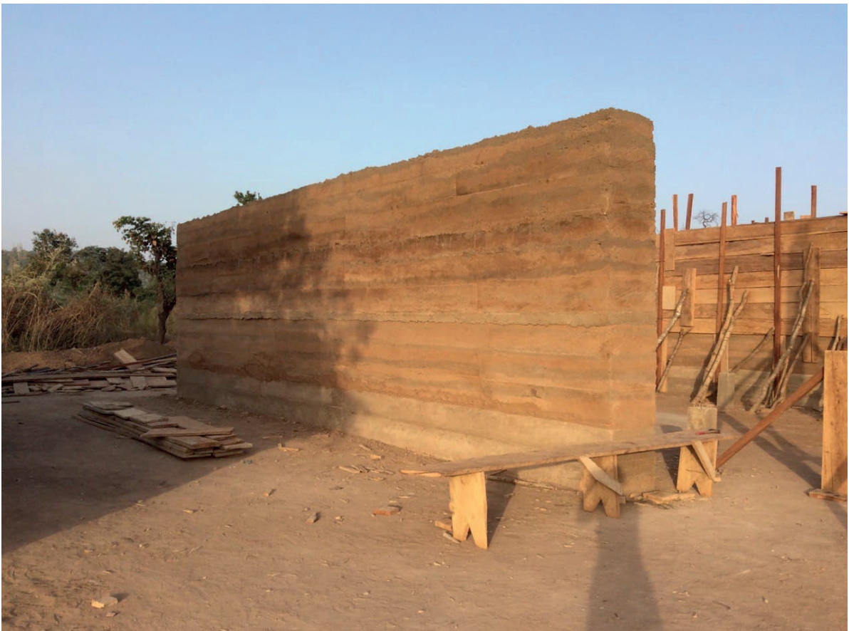
Figure 36 - Image of the construction process. Rammed earth walls
