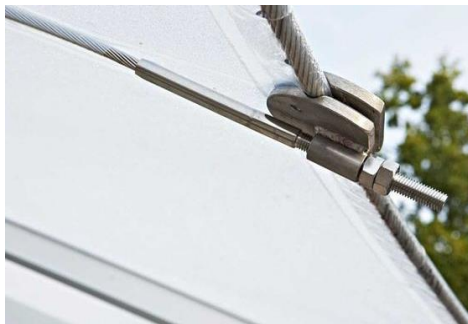
Figure 41. Direct tensioning with plate and prestressed rope [45].
