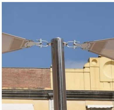
Figure 12. Tensioned to a support with two connections [12].
