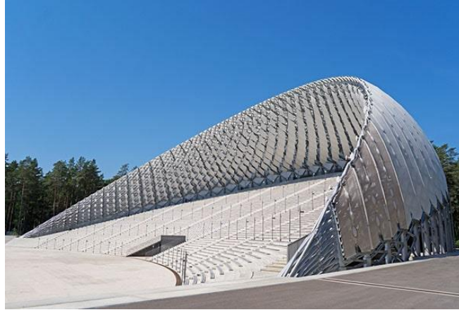
Figure 37. Grandstand Roof, Latvia [41]
