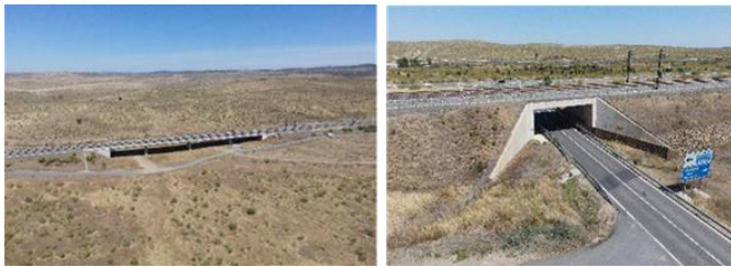
Figure 6 Demonstration project railway bridges
