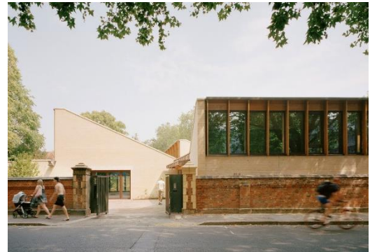
Sands End Arts & Community Centre – Mæ Architects
