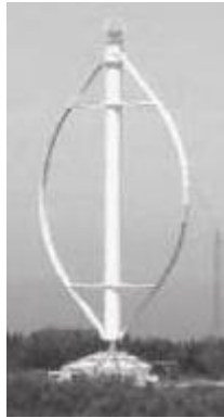
Illustration 25. 4 MW Darrieus wind turbine [20].
