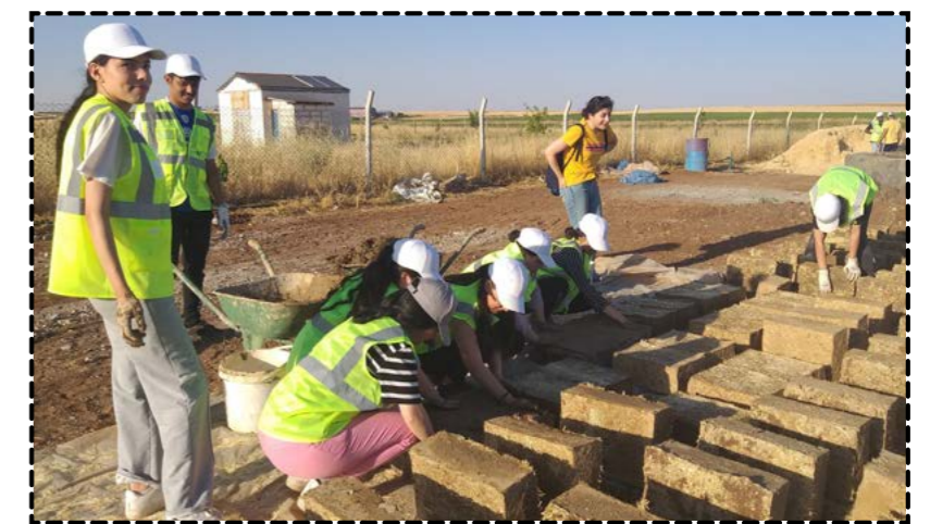
[Picture 30]. Adobe House construction, Ecotov
