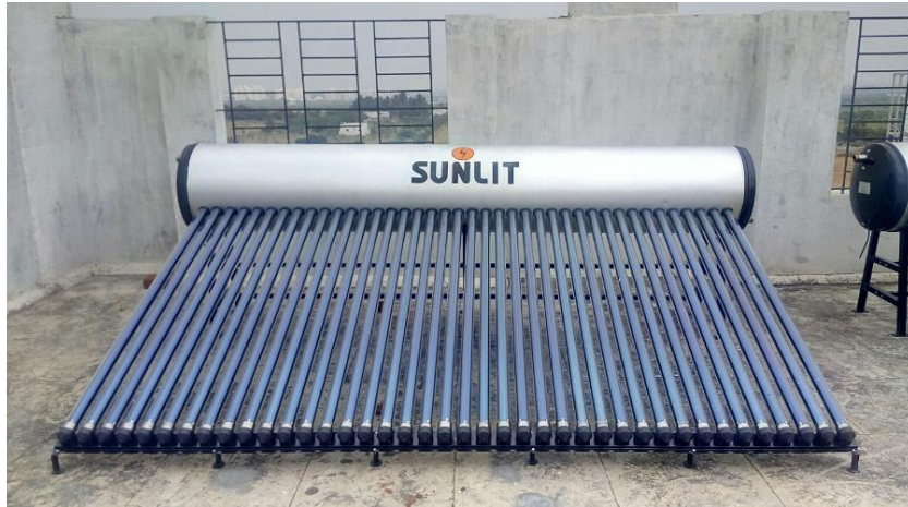
Figure 4. Example of evacuated tube collectors. (Source: Innergy.com)
