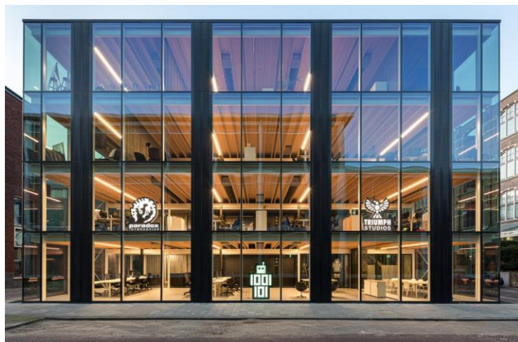
Figura 115. Fachada (ArchDaily, Ma.Francisca González, 2020).
