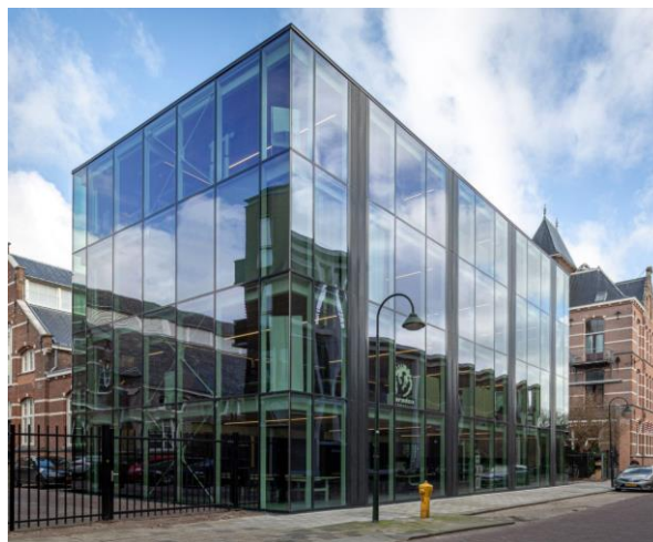
Figura 116. Fachada (ArchDaily, Ma.Francisca González, 2020).
