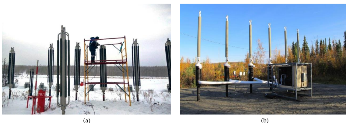
Figure 1. a) vapor-liquid thermostabilizer recharging with refrigerant [25], b) refrigeration machine connected to soil thermostabilizers [22]
