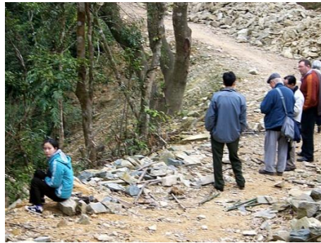
Ecotourism road construction through the Camellia petelotii site (2007)
