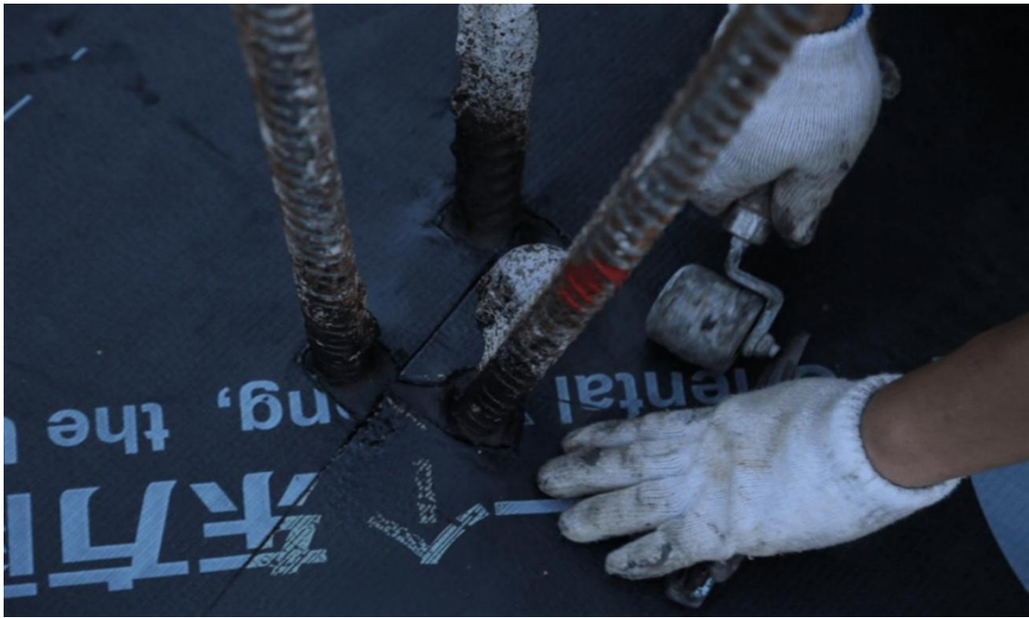
Figure 5.11 Oriental Yuhong construction site
