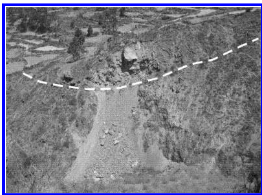
Figure 5. Dashed line indicates the contact between a coarsely jointed andesitic flow unit and the underlying pervasively fractured red tuff unit. The slope is about 70 m high. The rockfall occurred within the past 20 years and continues to grow as the failure in the red tuff undermines the andesite flow. Bouldery debris from the rock fall blocks the channel of Payhua Creek.
