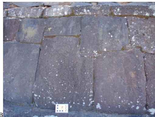
Fig 5. Interlocking techniques used in Cusco (picture: Arturo Oliveros) (A) and in Tzintzuntzan (B)
