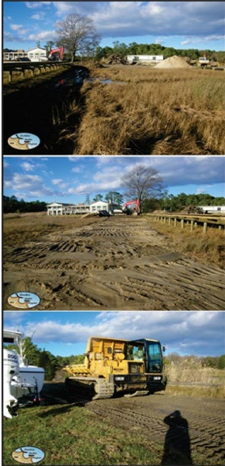
Figure 5-13. Photos taken during construction at Captain Sinclair's Recreational Area on 29 Jan 2016.
