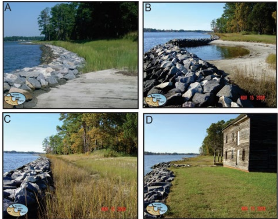
Figure 4-5. Sill system at Poplar Grove on the East River in Mathews County, Virginia six years after completion. A) The sill and marsh fringe provide a wide buffer between the water and the upland. B) The wide gap in the sill provides a pocket beach access area along the shoreline. C) The project zones are clearly visible: stone sill, S. alterniflora , S. patens , and upland/wooded. D) The old mill sits close to the shoreline. In this area, a revetment was chosen to protect the shoreline.
