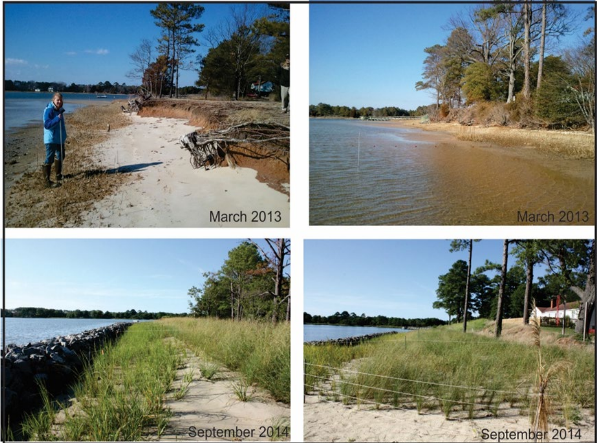
Figure 5-6. Occohannock on the Bay shoreline before (top) sill construction and after (bottom) construction.
