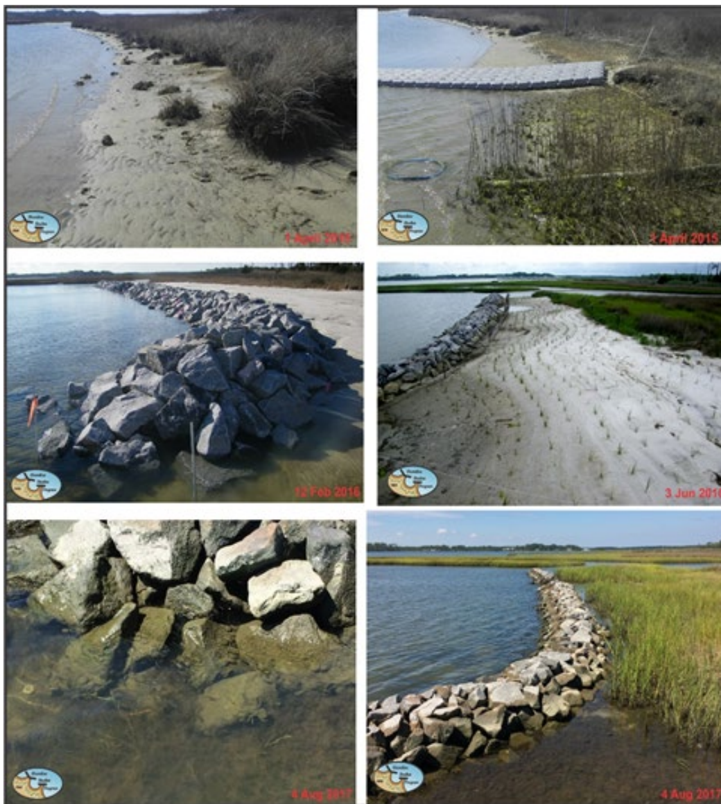
Figure 5-10. Captain Sinclair's Recreational Area pre-construction (top), post-construction (middle), and a year later (bottom). The marsh grasses are lush, SAV has grown behind the structure, and fauna are utilizing the rocks and the marsh.
