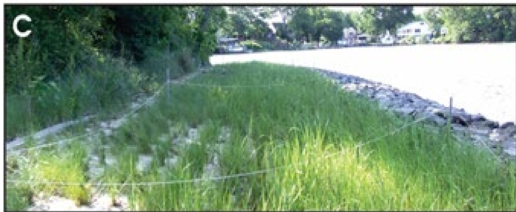
Figure 4-9. Hull Springs Farm shoreline A) before construction, B) after construction of the sill and placement of sand, and C) after planting.
