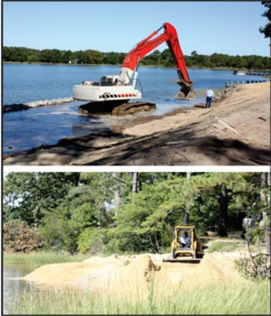
Figure 5-5. Construction of the shore structures at Occohannock on the Bay.
