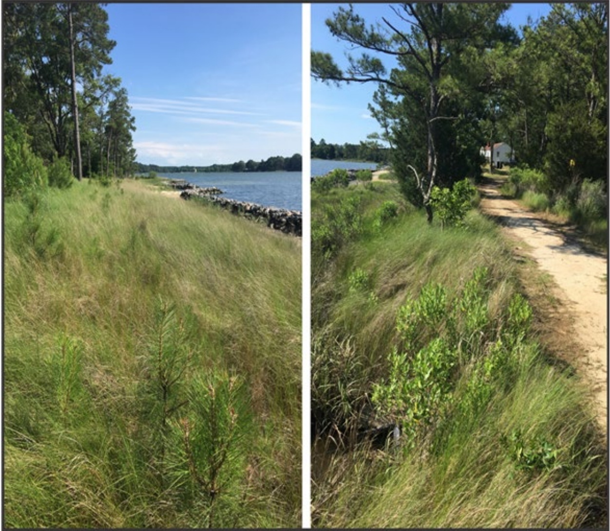
Figure 5-7. Photos of the project three years after installation in May 2017. The marsh behind the sill is expansive (left) and the access road is no longer threatened (right).
