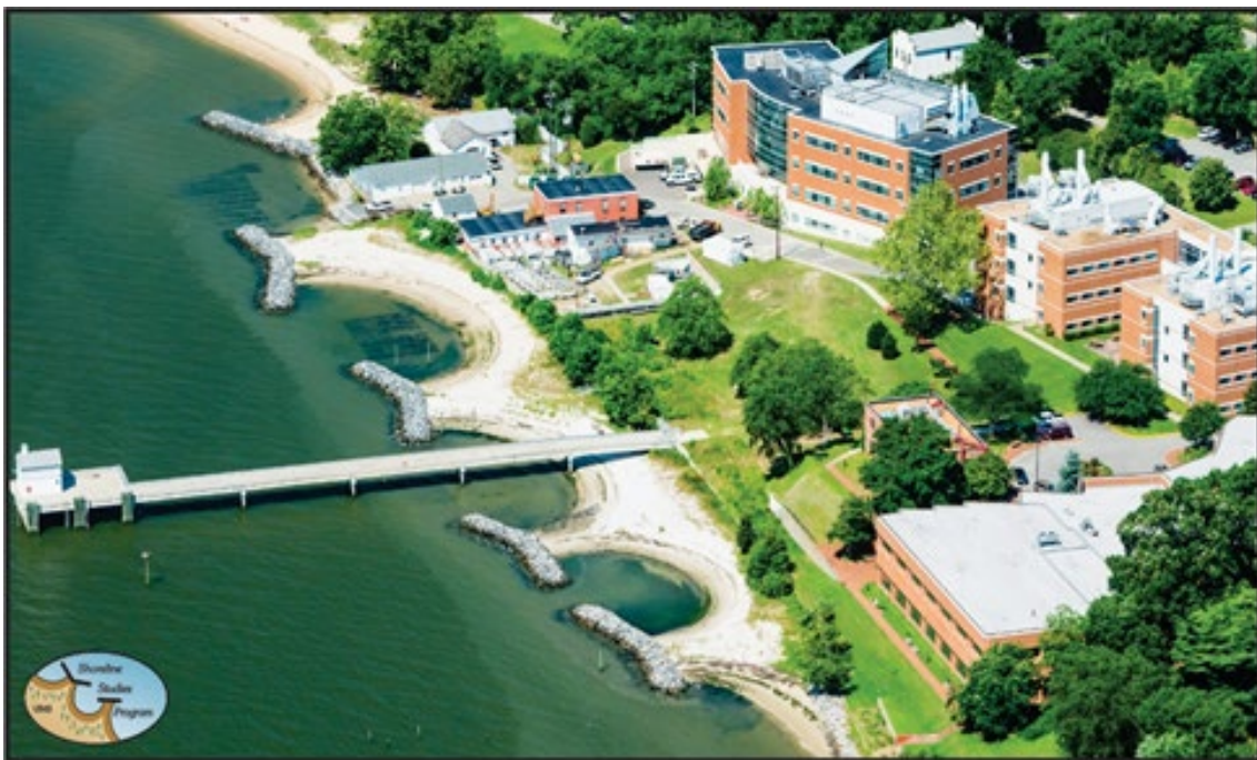
Figure 3-8. Aerial photos of breakwaters at the Virginia Institute of Marine Science campus on the York River. While the physical characteristics of breakwater sites differ, the goals are the same: protect the upland bank/marsh with a wide recreational/ protective beach.
