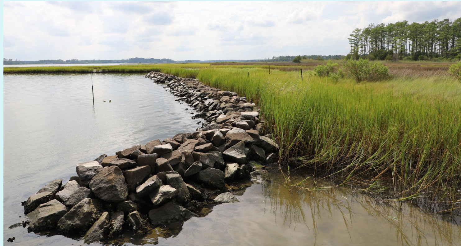
8 years post-installation (August 2023)
