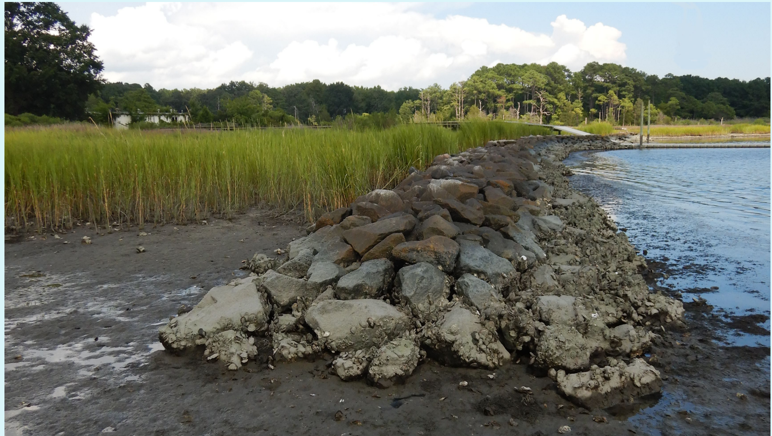
7 years post-installation (August 2022)
