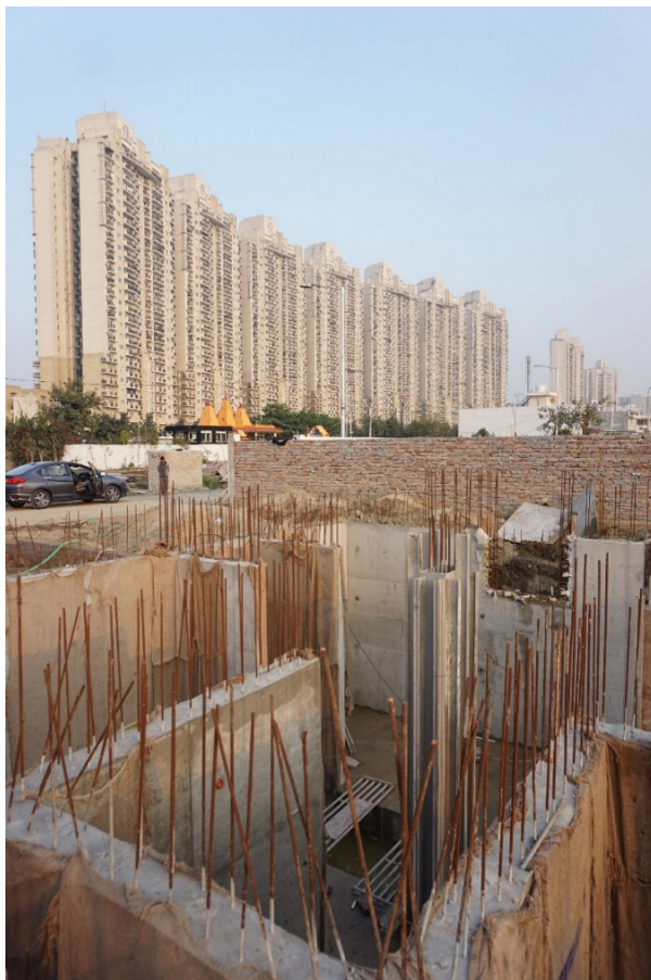
Figure 1: Construction of multi-story concrete housing outside of New Delhi, India.
