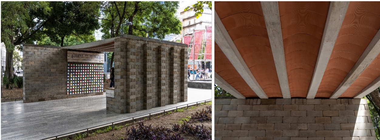
Figure 11: Sueños con tierra, a constructed pavilion with a close-up view of precast shaped beams supporting 3D-printed clay blocks that serve as lost formwork for a cast-in-place topping slab. Photo by Walter Shintani.
