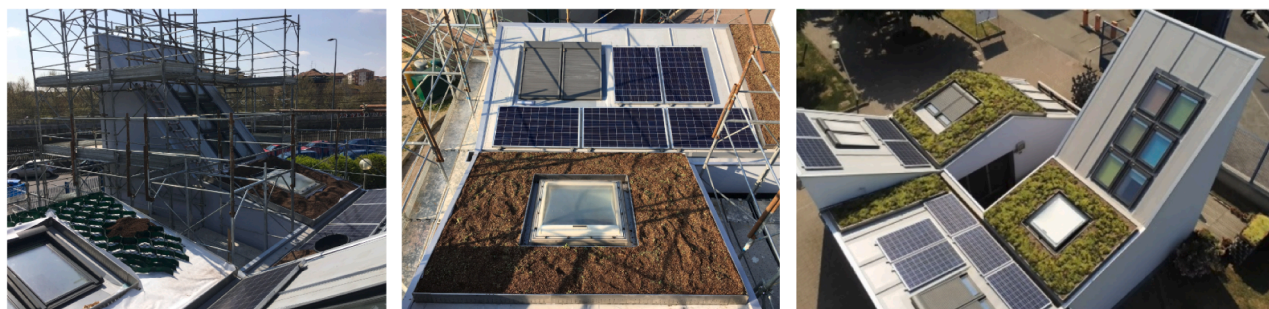
Fig. 19. Schematisation of the lightweight green roof system installation. (For interpretation of the references to colour in this figure legend, the reader is referred to the web version of this article.)
