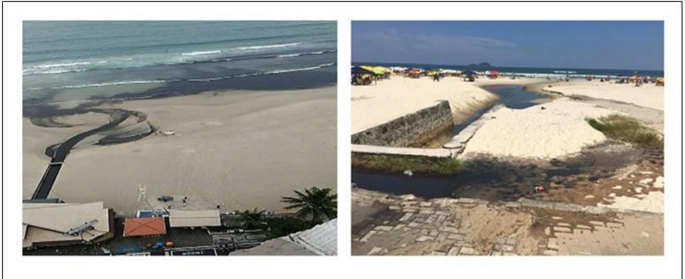
Figure – 1.11: Municipality of Guarujá, State of São Paulo: accidental sewage leak in Pitangueiras beach (2018), conducted to the sea through urban drainage channels.
