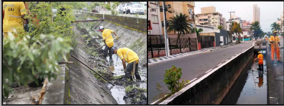
Figure - 10.3: Services of silting (a) and cleaning (b) performed by the city hall of Guarujá in the urban drainage channels of Enseada, Guarujá, Brazil.
