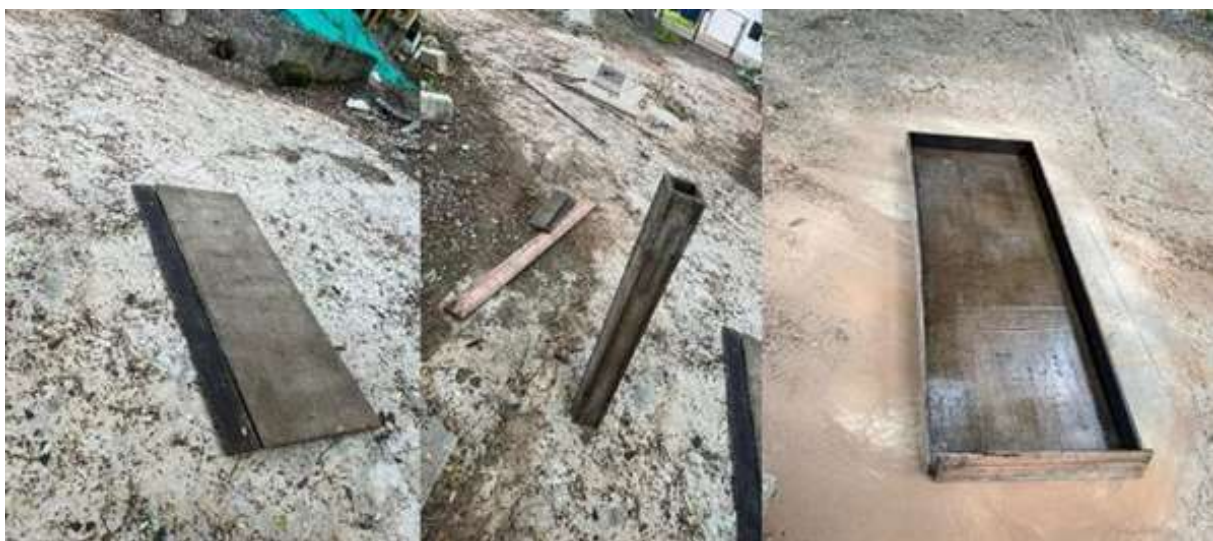
Figure 5. Plywood formwork painted with oil
