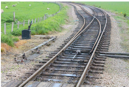
Figure 5.6: Point at Broomhill station, Scotland. Licensed under the Creative Commons Attribution-Share Alike 4.0 International license [117].
