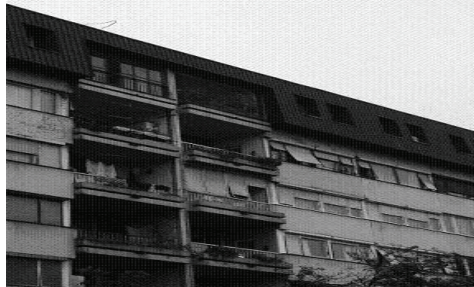
Figure 2. Typical south-west facade
