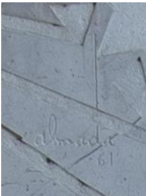
Figure 11. Example of Almada's signature in the façade of the rectory of the University of Lisbon. Photo: Telmo Domingues.
