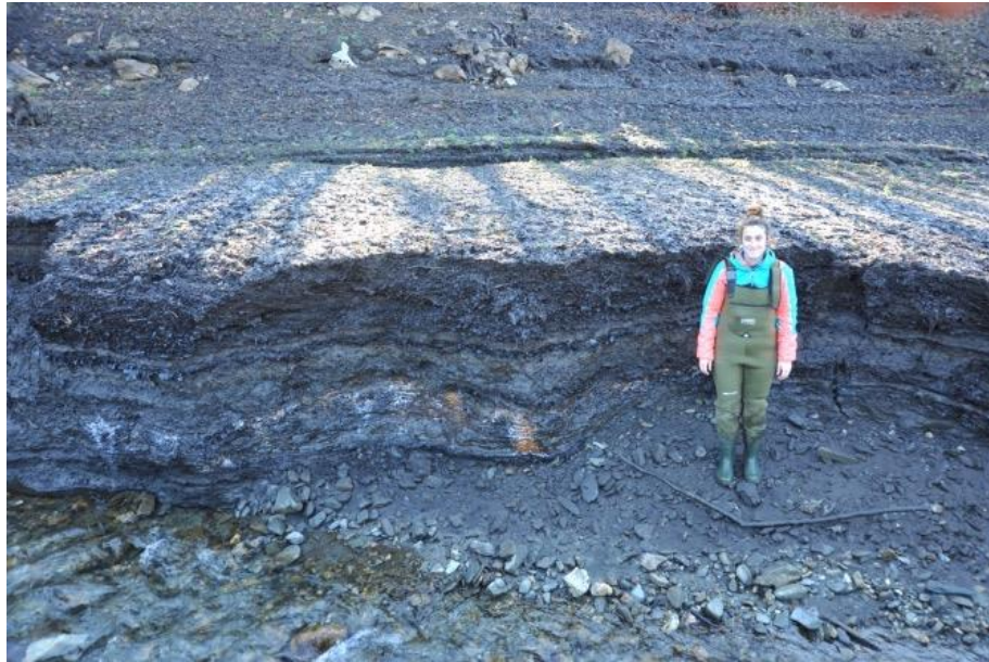
Figure 4.1.2. Detailed photo of the riverbank excavated by the Enobieta Stream in the reservoir tail area. The terrace is made up by discrete layers of leaf litter, silt and clay, and gravel. Note iron precipitates in the bottom part. Picture: Arturo Elosegi.
