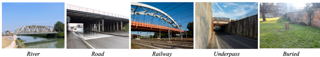
Fig. 13. Examples of bridges spanning various types of obstacles, observed in Padova inventory.
