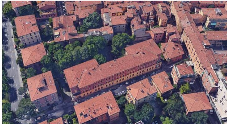
Figure 1: The elementary school G. Pascoli in the centre of the picture
