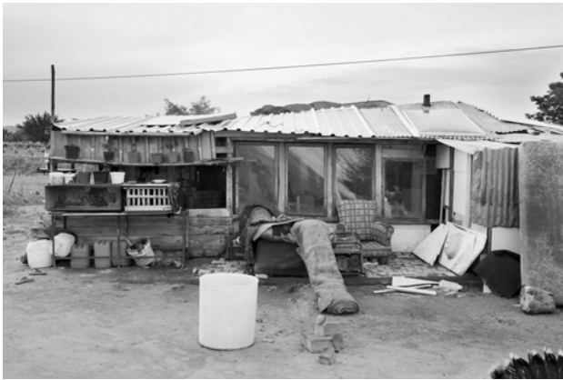
Figure 7.9: Makeshift vineyard shed in Ürgüp
