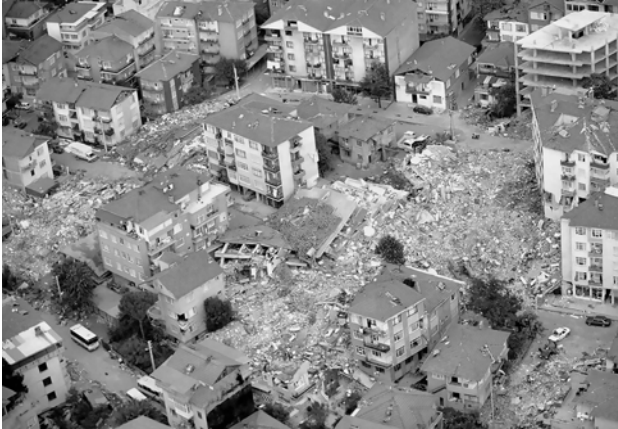
Figure 4.11: The destruction caused by Izmit earthquake in 1999
