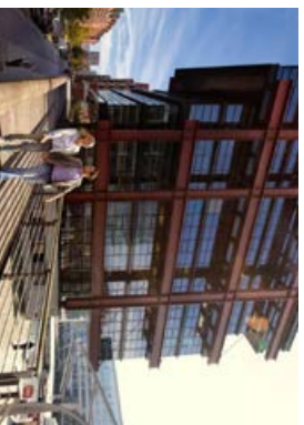
FIRST FL. ON THE PROMENADE SEALS OFF FOR FLOOD BLDG BEHIND PROMENADE BUILT ON "TERPS"
