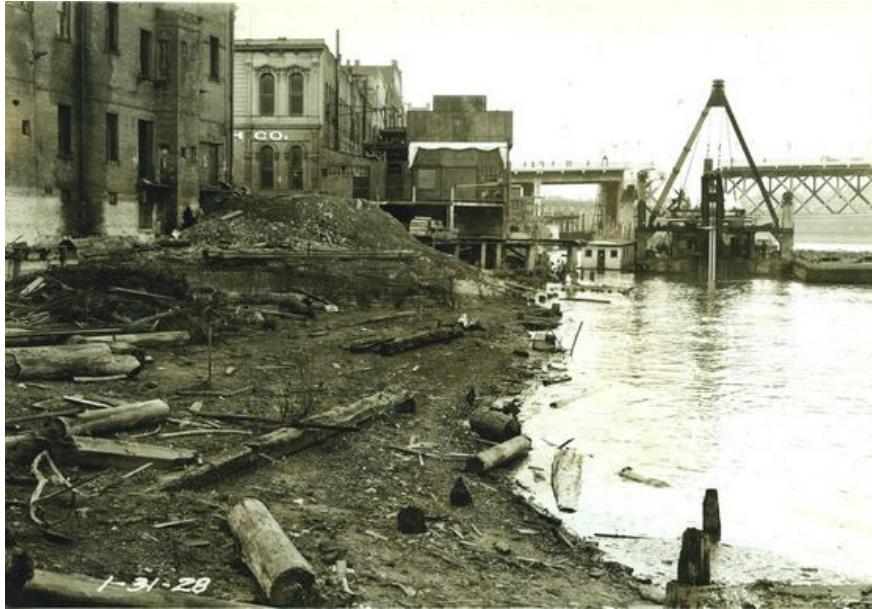
1928- Portland's West Side Waterfront Construction
