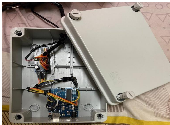
Figure 3.4 2 Shows the electronic components fixed in the power box
