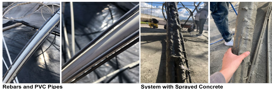
Figure 3. System Implementation with Concrete
