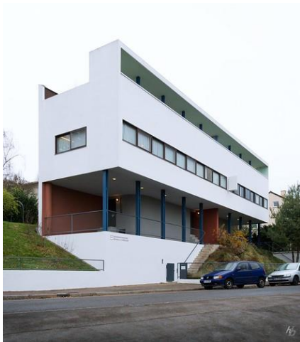
Figure 27:The two-family structure known as Houses 14 and 15
