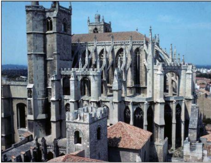
Figure 52: Narbonne Cathedral Exterior with Buttressing
