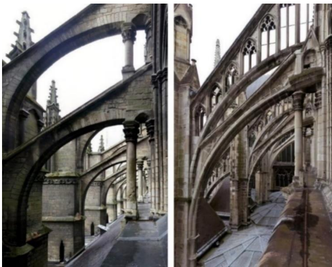
Figure 51: Flying buttresses at Amiens Cathedral
