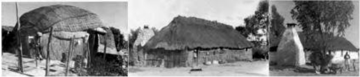
Figure 10: Vernacular Architecture of the Cape. Left: A circular matjieshuis, Middle: Rectangular reed-walled cottage, Right: reed-walled cottage,
