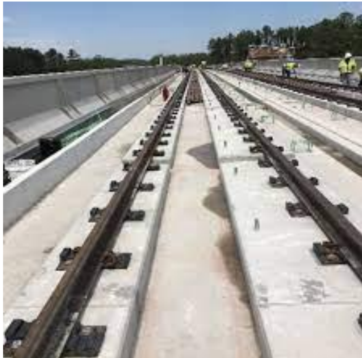
Figure 2-5: Direct Fixation Deck (Kim et al. , 2019).
