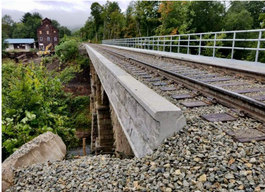
Figure 2-4: Ballasted deck (Riley, 2018).
