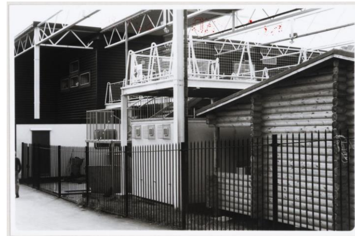
Figure 62 Exterior view of InterAction Centre.
