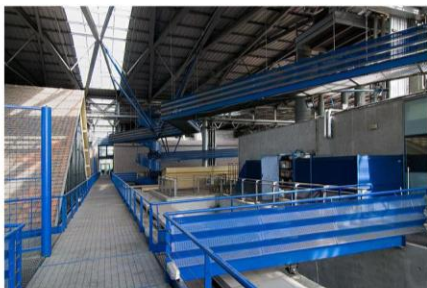
Figure 71 View on walkways in in-between space
