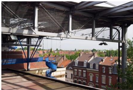
Figure 70 Girder truss spanning between large columns
