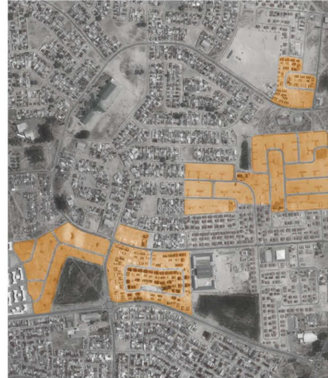
Figure 60 Open land parcels prepped for the construction of housing, image edited by the author, base image sourced from google earth, 2022
