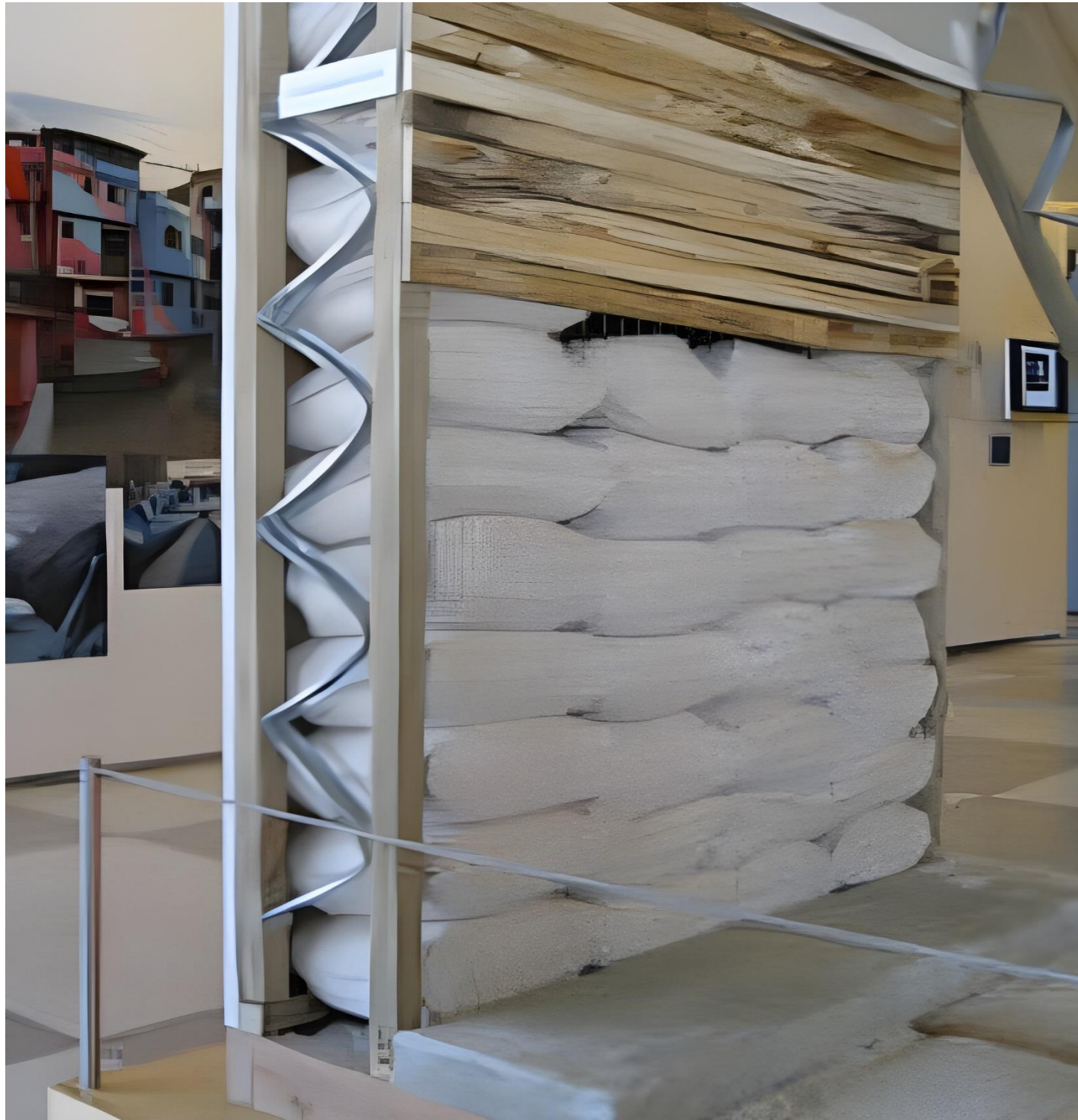
Figure 12 Sectional models showing the tectonics of a sandbag wall. (Engineering For Change. 2022. )
