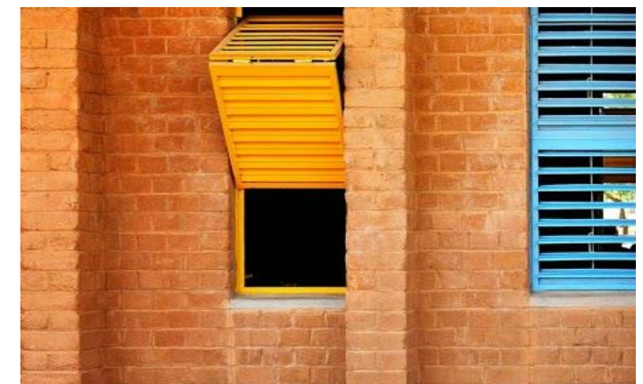
Figure 11 Steel shutters made by local steel craftsman in Gando. (Ouwerkerk, E., 2016.)
