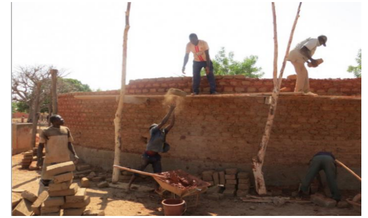
Figure 5 Construction of the mudbrick walls. (Design Indaba. 2022.)
