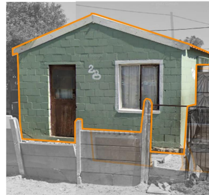
Figure 54 The use of concrete blockwork in the construction of buildings (by the author, 2022)
