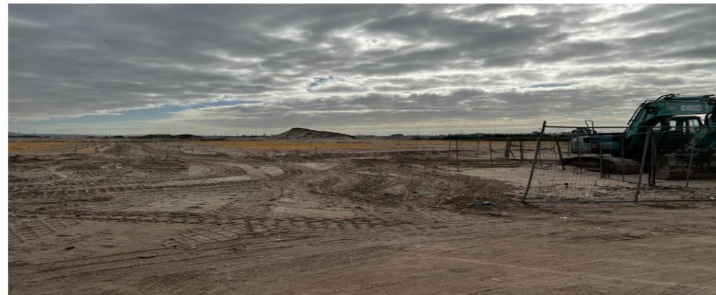
Figure 62 Image of the site under construction (by the author, 2022)
