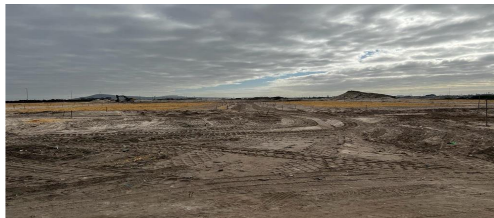
Figure 63 Image of the site under construction (by the author, 2022)
