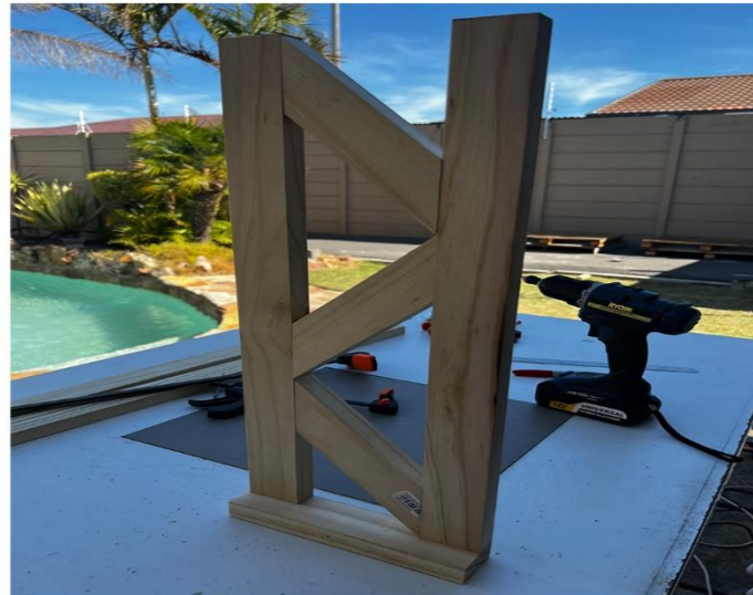
Figure 14 Completed timber ladder (By Author, 2022)
