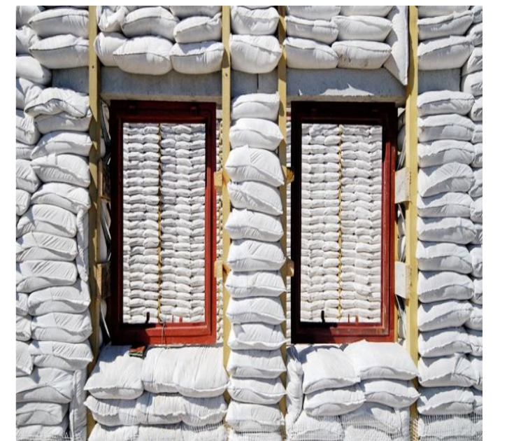
Figure 24 Exposed construction of a sandbag wall (yakhahuis, V., n.d.)
