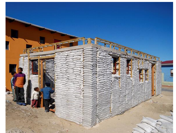
Figure 25 Completed the first storey of a sandbag structure (Archigraphy.com, n.d.)
