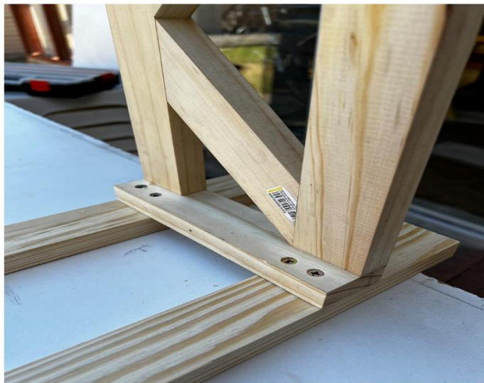
Figure 15 Fixing the timber ladder to the base (By Author, 2022)
