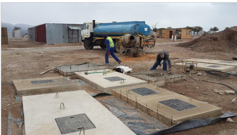
Image O: Drainage systems put in place for area 4C (Aurecon, 11/28/2013).
