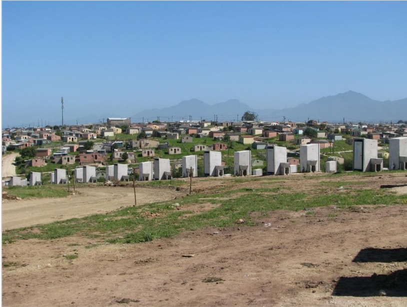
Image M: Row of enhanced serviced sites, i.e. provision of each household of a toilet and standpipe (Aurecon, 11/28/2013).
