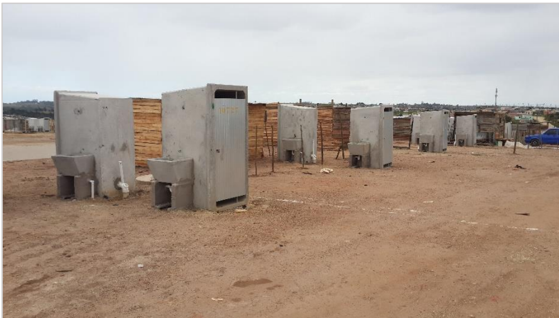
Image N: Closer view of enhanced serviced sites. Residents either built over these serviced sites, or, as this picture shows, how the toilet - standpipe unit is outside, and the informal structure is built in front of it. (Aurecon, 11/28/2013).
