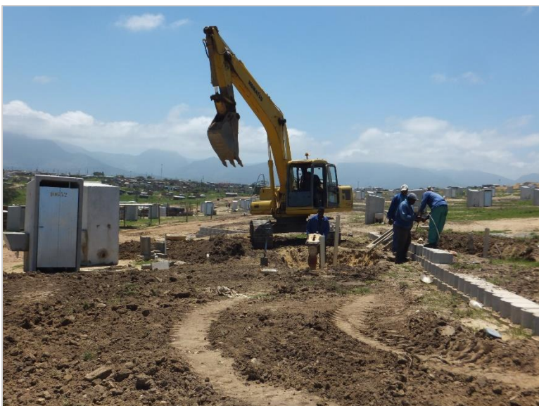
Image L: Machinery used in preparation for infrastructural provision (Aurecon, 11/28/2013).
