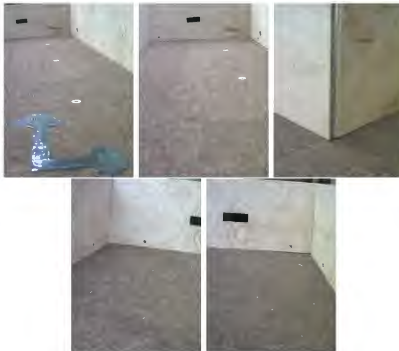
Figure 5.6: Images of the Duct Using the Forward Facing Camera
