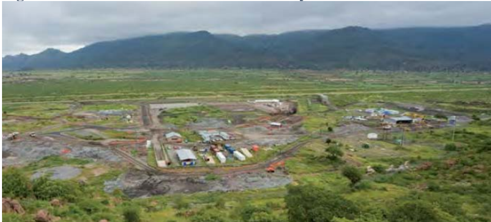
Figure 21 - A view of Twickenham's Hackey Shaft
