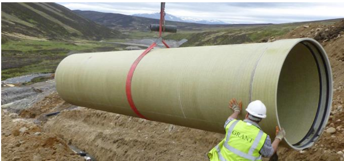
Figure 2-49: A GRP pipe being slewed into position (GRANT, 2016)
