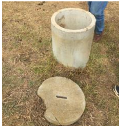
Figure 5-48: Air valve concrete chamber
