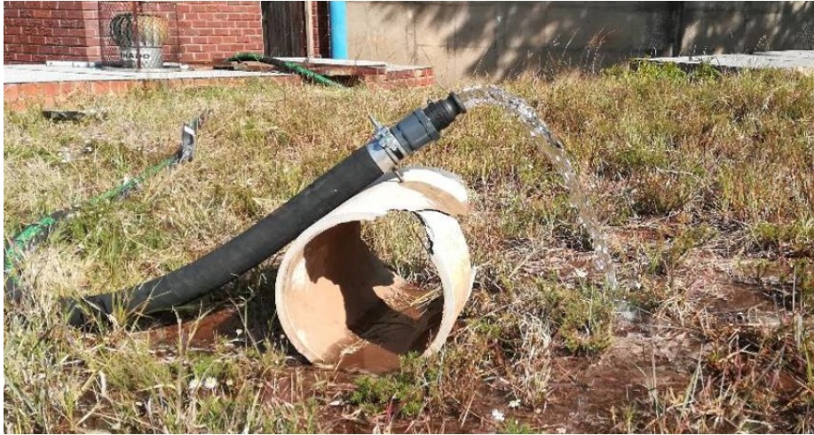
Figure 5-14: Constant flow observed after both valve AV1 and V2 were closed
