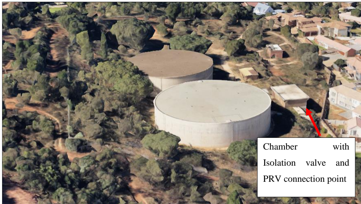
Figure 5-3: Google earth image of reservoir configuration
