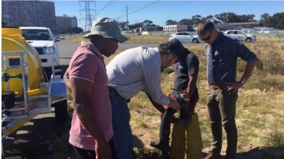
Figure 5-69: Shows the PCAE 50mm hosepipe being connected to the fire hydrant
