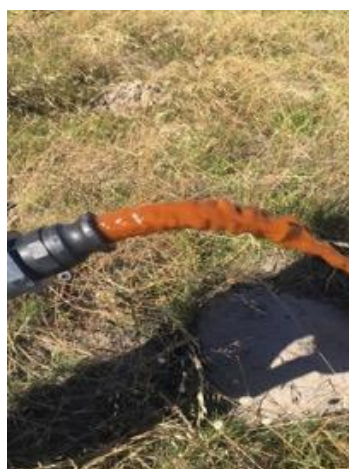
Figure 5-70: Showing the colour of water during flushing
