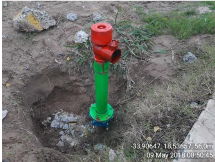
Figure 5-83: Replaced fire hydrant pipe and head
