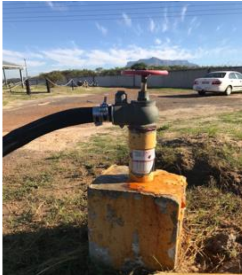
Figure 5-86: Installed fire hydrant head with the PCAE Connected
