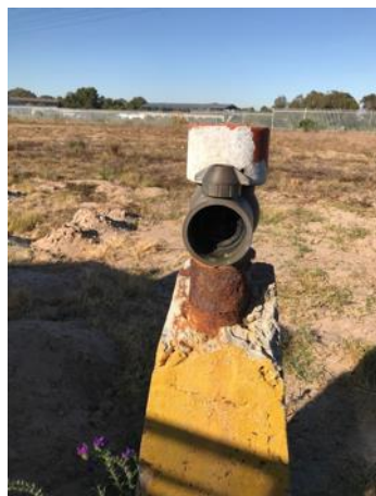
Figure 5-81: Fire hydrant connection
