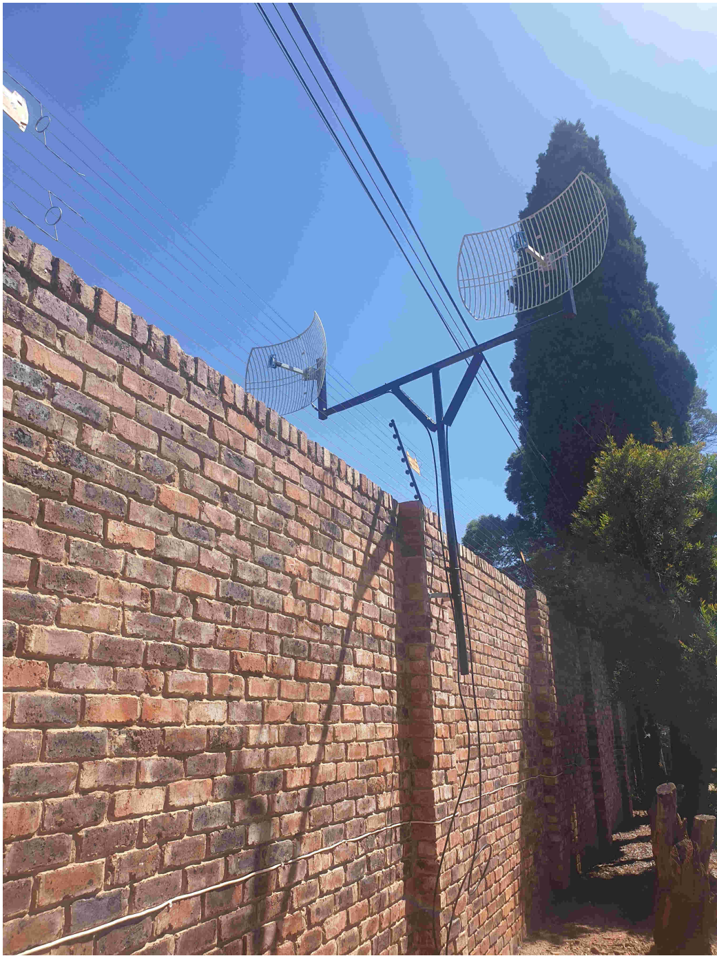
Figure 5.9: Antenna Setup For Car Detection
