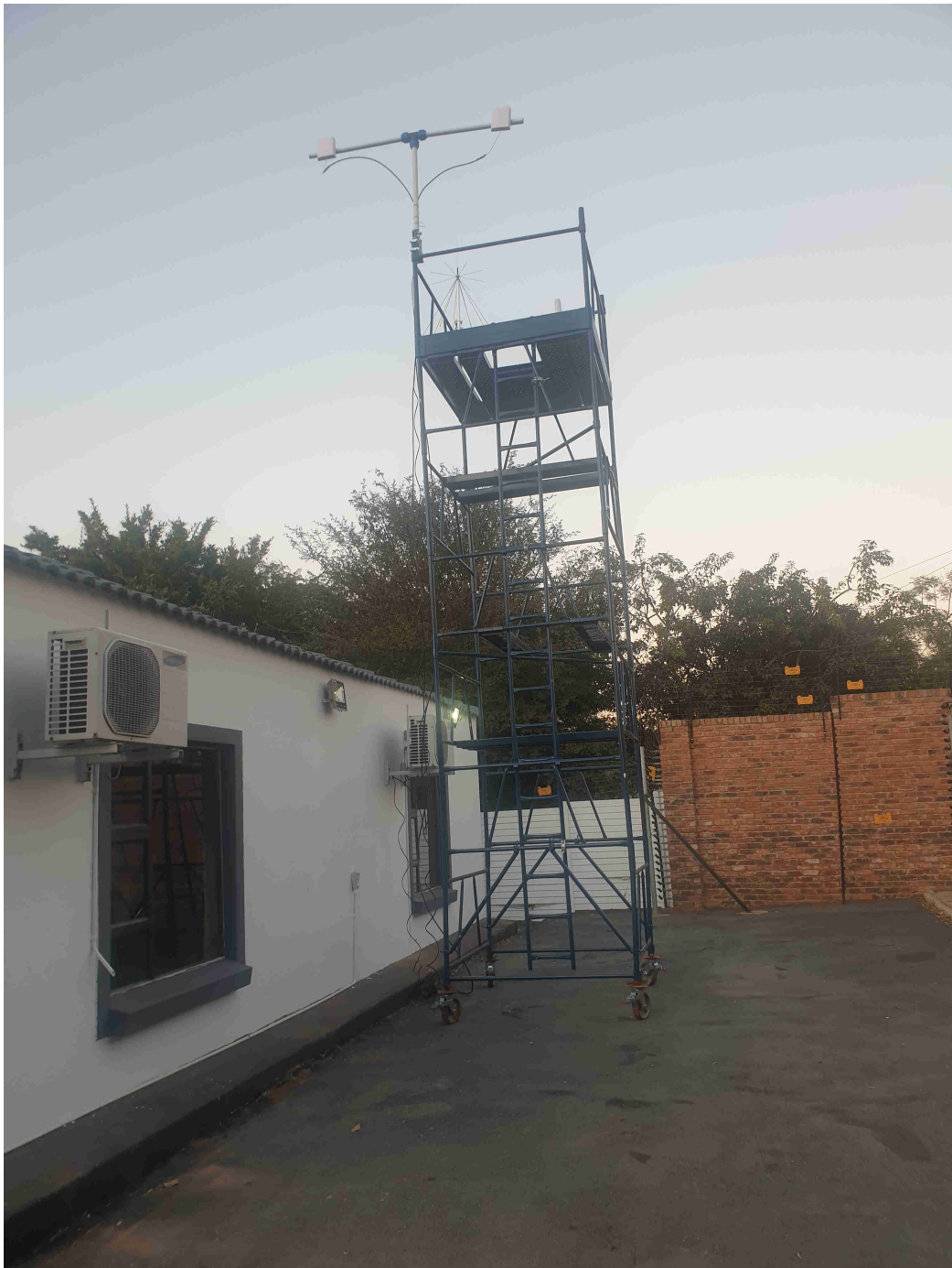
Figure 5.19: Antenna Tower Deployed For Airborne Targets Detection Phase 2
