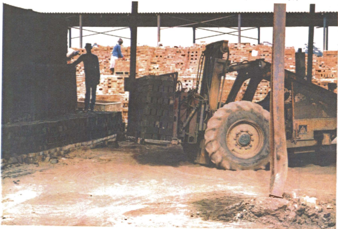
A Bell forklift approaching the clamp.
