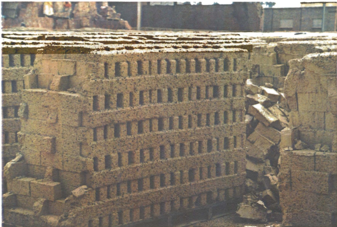
Partially damaged Mc Donald Pallets at Joostenberg Brick
