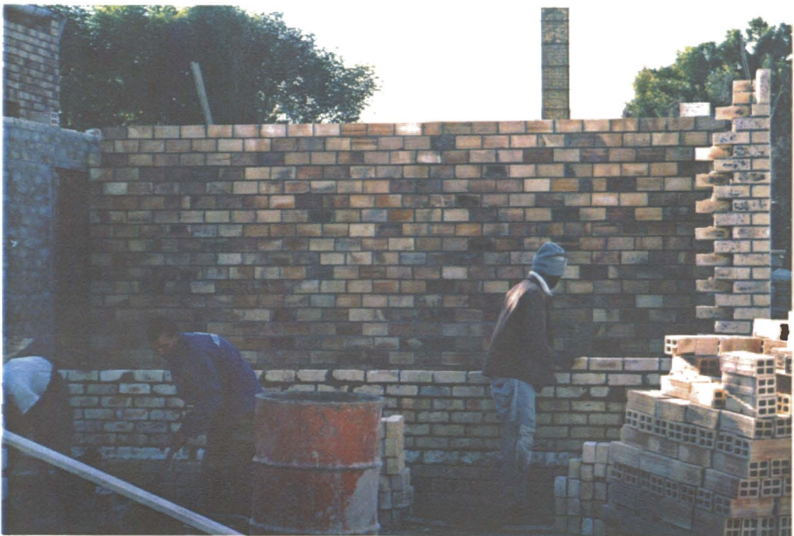
The WB4 being used as a Face Brick in an internal wall.
