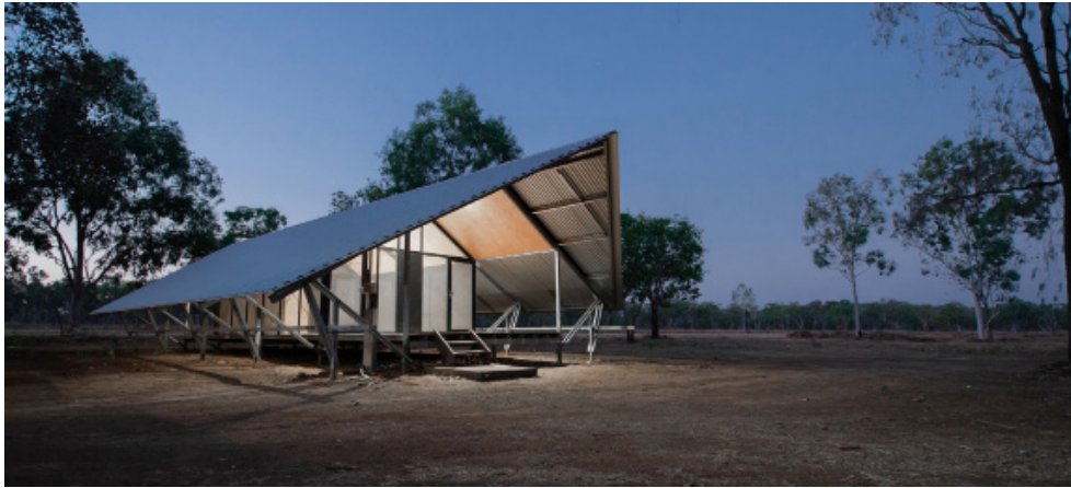
Figure 1: Fish River Aboriginal Ranger Accommodation, designed and built with students by the Design Construct programme (Joti Weijers-Coghlan 2017).
