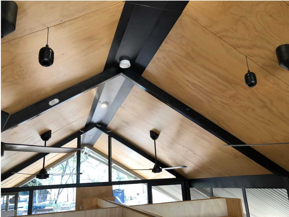
Figure 10: The installed thermal sensor network in the retrofitted accommodation (UniSA 2018).
