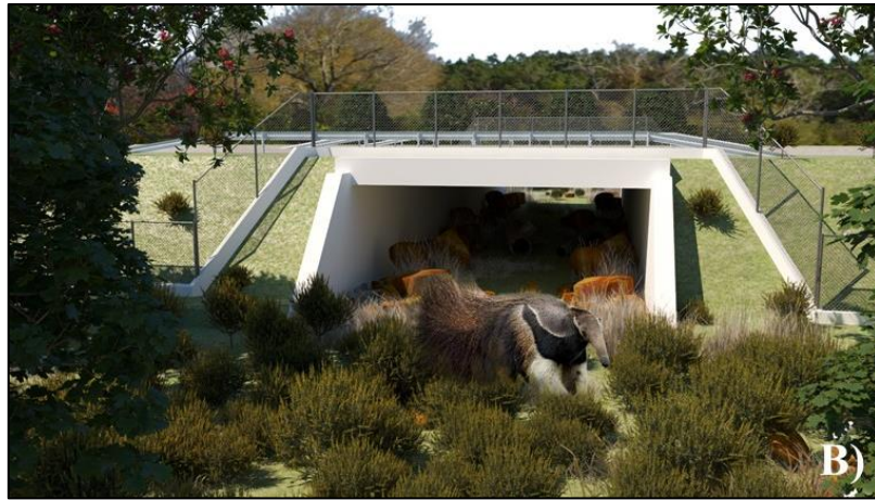
759 Figure S3.1 – The design of fence projected as a mitigation to decrease WVC (A), and in 760 combination with wildlife underpasses, water culverts or cattle boxes (B). Source: 761 ViaFAUNA Environmental Studies.
