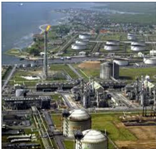
Fig. 1. Kaduna Refining and Petroleum Company
