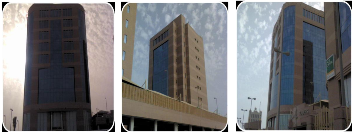
(a) Eastern façade
