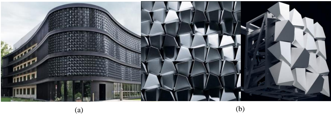
(a) A building with flare mounted. (b) The façade and a Flare showing 16 detailed flakes (components).
