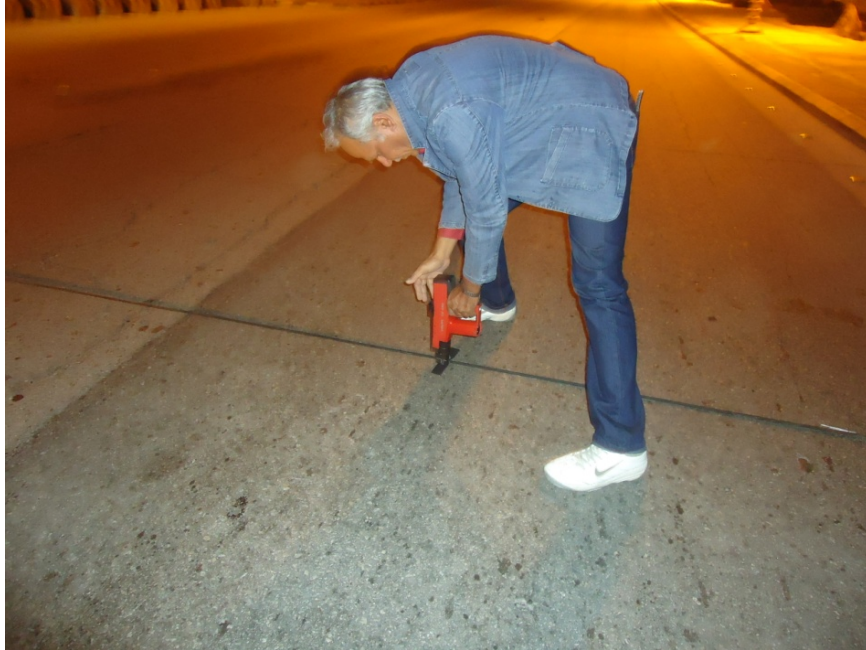
Figure 4-8 Embedment of pneumatic tube on the street.
