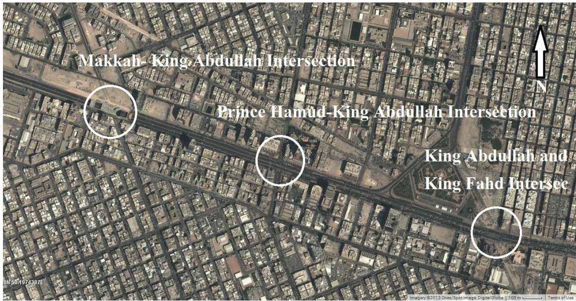
Figure 4-2 Aerial photograph of Study Area (Photo source: Google Earth Satellite image)
