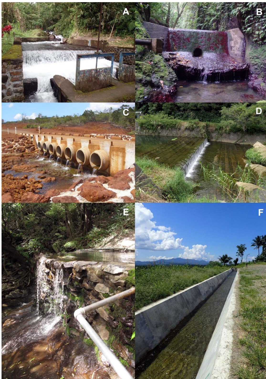
Figure 4. – Examples of heavily engineered human structures that modify short-steep-coastal-streams other than large dams. A: A fishway on a tributary of the Aling Aling River, Bali (Photo: PK); B: A concrete weir in Futuna (Photo: PK); C: Road crossing at Routes de sud, New Caledonia (Photo: CL); D: Concrete steps in Okinawa (Photo: KM); E: A small weir and water offtake to supply public toilets at Ellis Beach, Australia (Photo: BE); F: A straight linear concrete realignment of a creek in New Britain (PNG (Photo: CL)).
