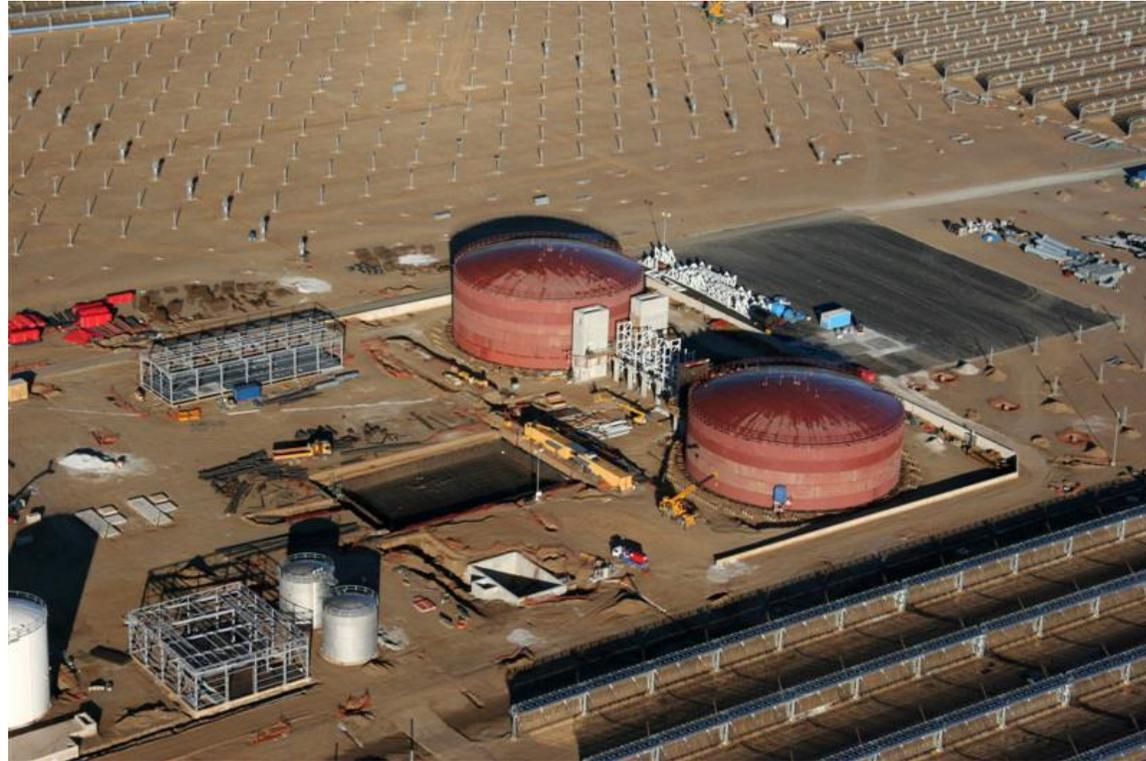
(about 30.000 tons of molten salt for 8 hours of  $50\text{MW}_{\text{el}}$  production)
